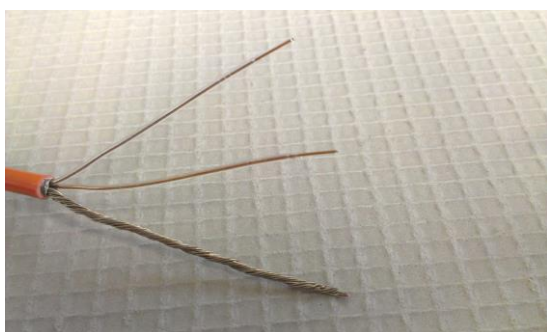
5) Stripped first end and then twist the Earth braid.
