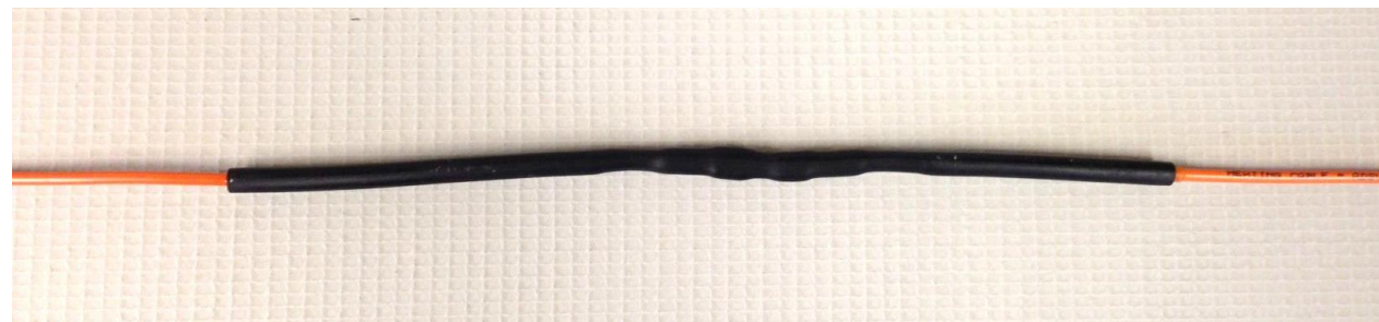
23) Finally slide the long Black sleeve so it is centrally over the repair and heat shrink in position. Allow the sleeving to cool down and check the resistance and insulation resistance between the live wires.
